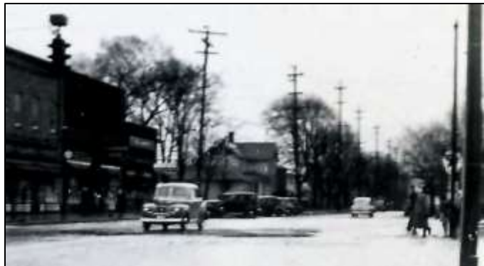
Broadway also had a light coating of flood water allowing traffic to pass.
