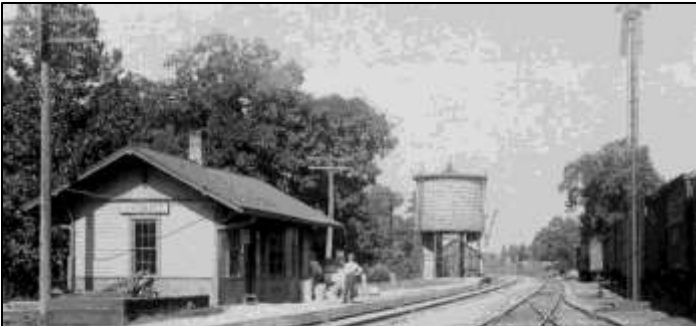
The Orient railroad station, originally known as Morgan's Station, was built in 1882.
